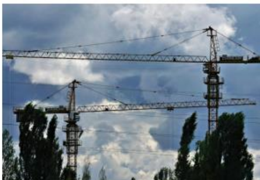
Figure 3: Cranes are especially vulnerable to lightning.
